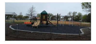
Eco-Turf installed the first layer of the poured-inplace surfacing at Jefferson Playground this week. They were not able to complete the project due to the much needed rain but will return next week to place the final red surface layer.
